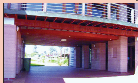
Figure 9 – The use of wide-span lintels with SRE walls at The Charles Sturt University campus building, NSW, Australia (© Earth Structures Pty Ltd.)
