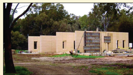
Figure 8 – The use of Stabilform™ to produce solid cavity-insulated SRE wall elements for a residential property in Benalla, Australia (© Earth Structures Pty Ltd.)
