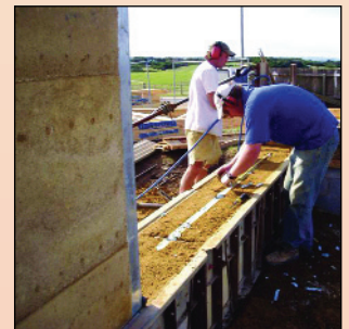
Figure 12 – The construction of an SRE wall incorporating solid cavity insulation and stainless steel wall ties (© Earth Structures Pty Ltd.)
